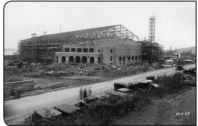
Construction was completed in 10 months, paid for mostly by $500,000 of funds from the Associated Students of the University of Washington.
