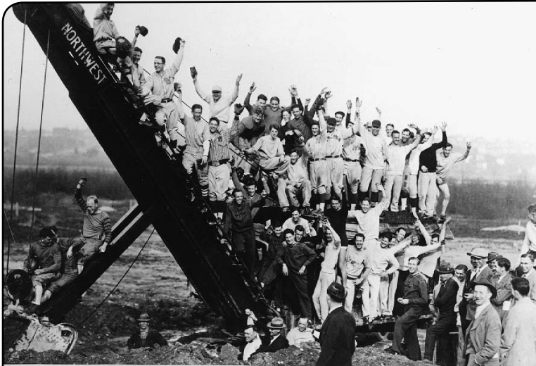
Ground Breaking for U. of W. Pavilion
